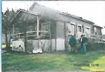
Ripple House #1, 45968 Albert Street, Crofoot Addition, Concrete
