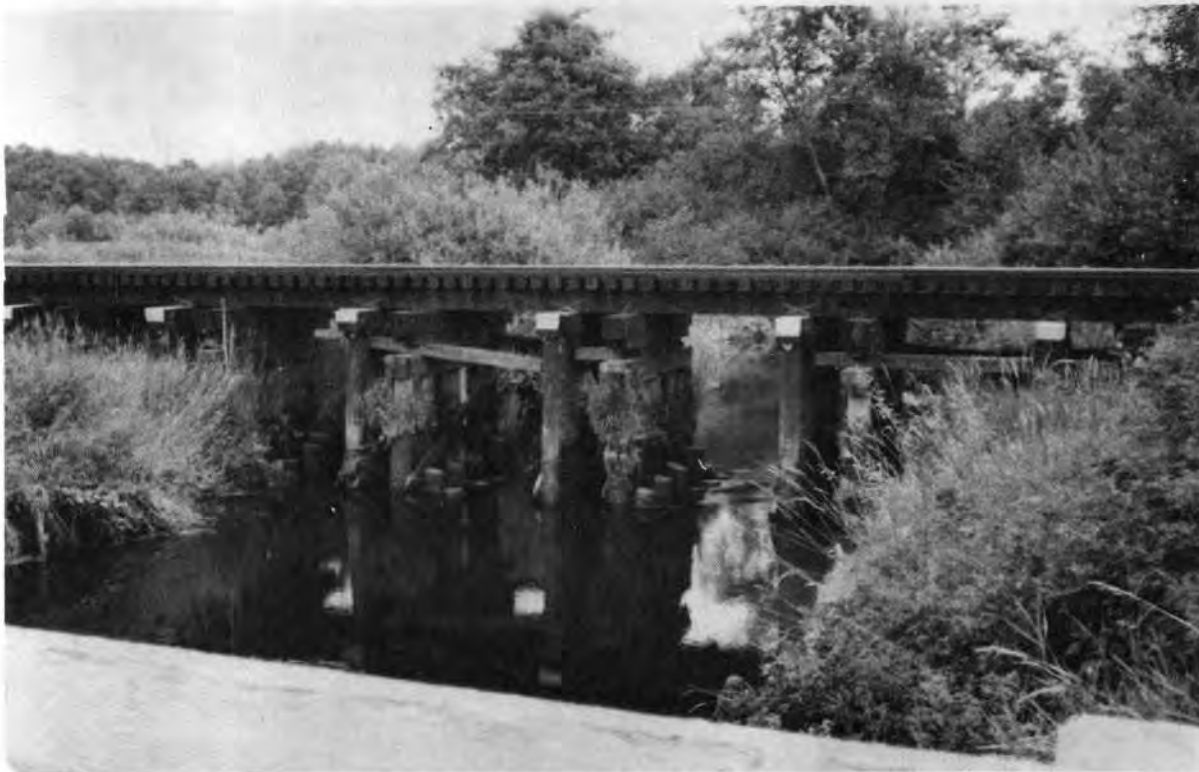
Photo 4-4. View west toward mouth of Fisher Slough where it flows into the Skagit River. Four hundred feet of the slough will be realigned to permit construction of the levee on the left bank. Right bank vegetation will be restored.
