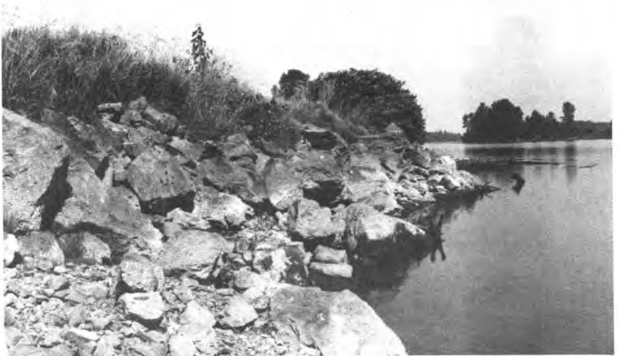
Photo 4-5. View of right bank, main stem of the South Fork during August low flow. Note that vegetation has reestablished within existing riprap down to the level of ordinary high water.
