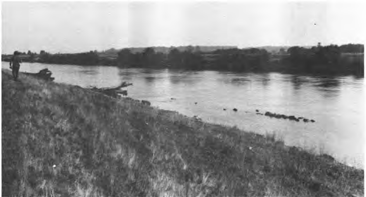
Photo 4-2. View of North Fork looking east at left bank, stations 100 - 120. Levee on the left bank will be adjusted landward to avoid removal of river-edge vegetation.
