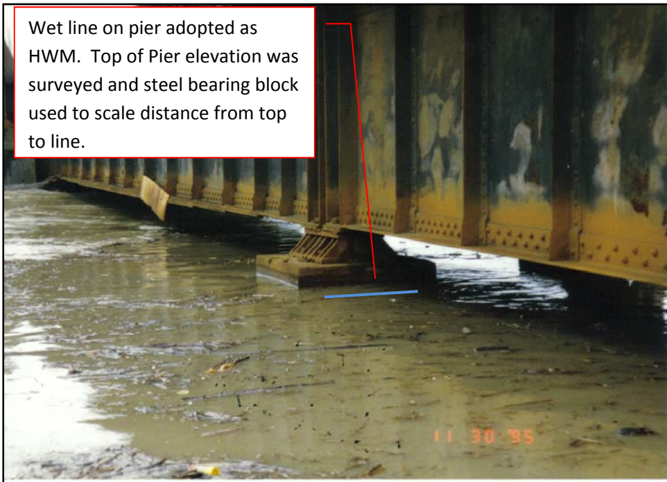
Figure 2-4: Close up of BNSF Bridge Pier during November 1995 flood
