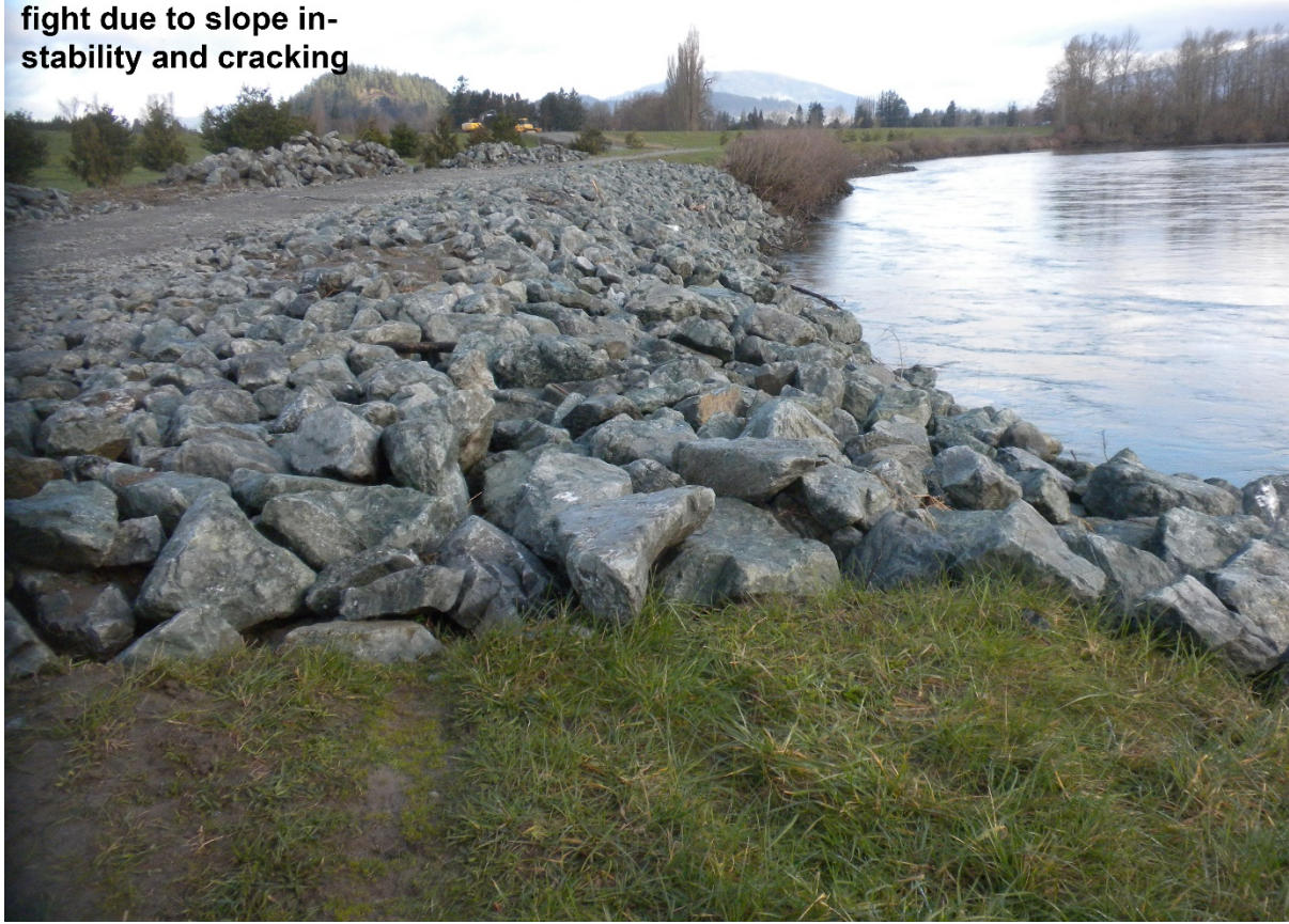
Figure 3. DD 12 300 LF flood fight segment looking upstream.
