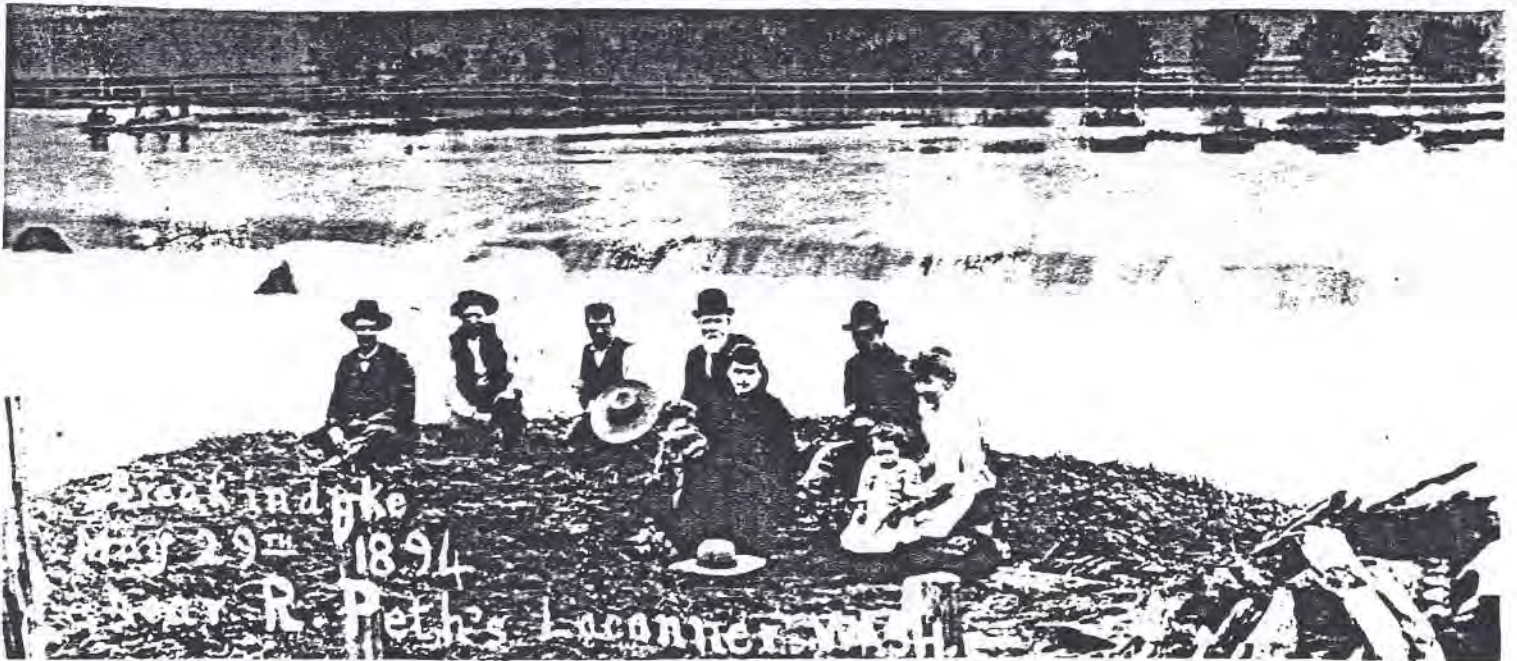
May 29th, 1894 flood at R. Peth's farm. The break is in the salt water dike. Current is water draining from land to the slough back into the bay. Notice there is no record of this flood provided by the federal government.
