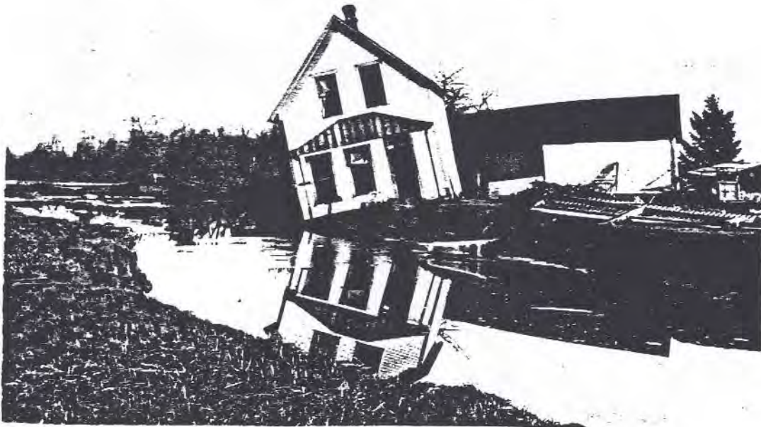
A classic example of what happens when you build structures next to conveyance areas. This house was located near what is now called Gages Slough.
