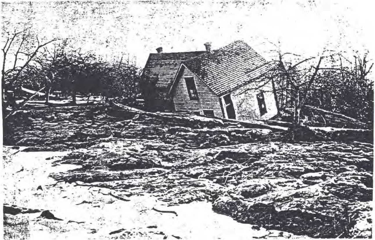
Nat Moore's house after the flood of 1909 which broke the dike between Mount Vernon and Avon. The house was located near the town of Avon.
