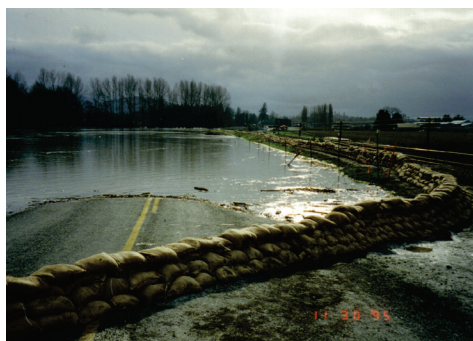
Sandbagging along Whitmarsh Road, Burlington Picture courtesy Dike District 12
