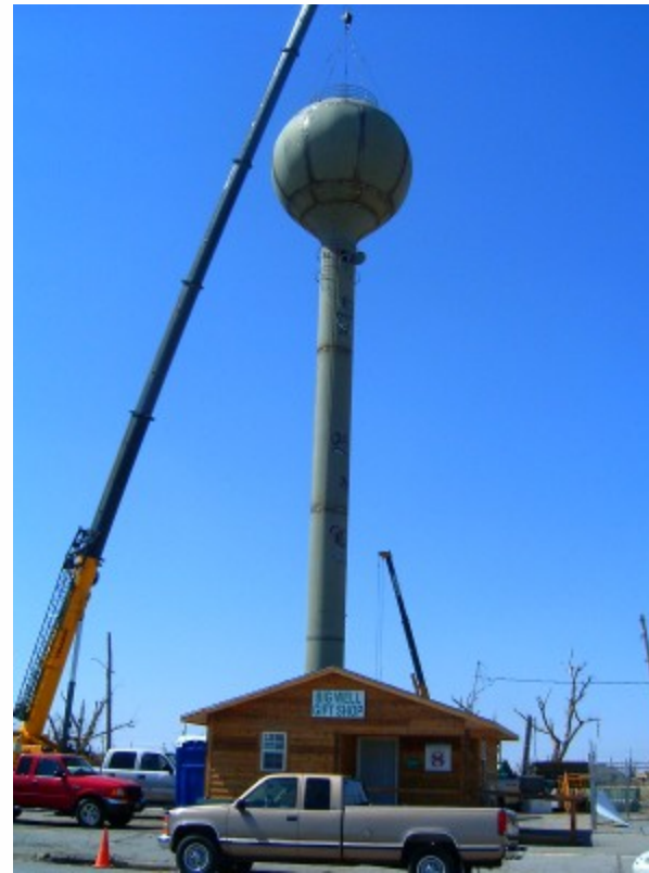
Water Tower in Kansas
