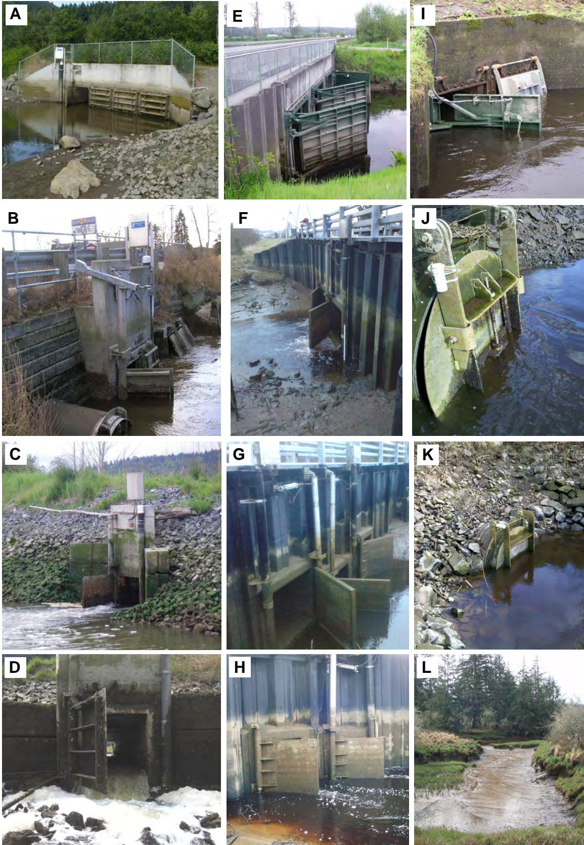
Figure 2. Self-regulating tide gates (A-J) and examples of a flap gate (K, North Hansen) and a reference site at low tide (L, Charlie Creek) used in the study design. SRTs are ordered from North to South as in Table 2. Photo credits to Jason Hall, except A (Brittany Jones), B (Oscar Bunting), C and E (Dana Rudy), D (Todd Mitchell), H (Kirsten Weinmeister), and I (Curtis Roegner).
