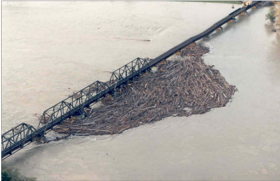
Army Corps of Engineers November 1995 Photo of the Burlington Northern Railroad Bridge
