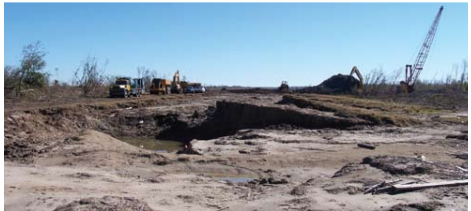
Levee Damaged Due to Overtopping Hurricane Katrina (August 2005) St. Bernard Parish, Louisiana
