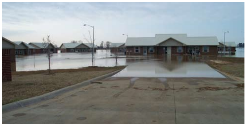
Flooding of Patrick Manor Senior Housing Community. Pocahontas, AR Photo by Elmo Webb, PE 3/23/08
