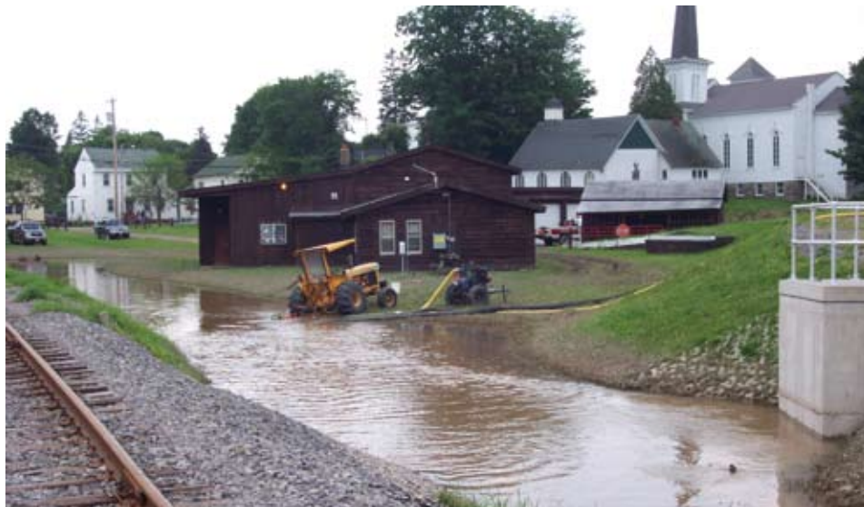
Floodfighting and Internal Drainage, Oxford, New York, 2006—Courtesy of NYSDEC
