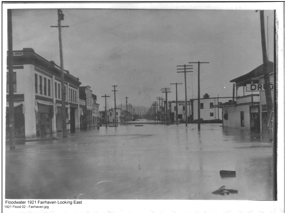
Fairhaven Avenue, Burlington, WA – Looking East (1921) (Courtesy of Roger Fox Collection)
