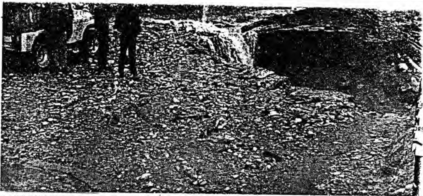
A ROAD WAS HERE —Grandy Creek Road gave way to the forces of rampaging water. This group of observers surveys
