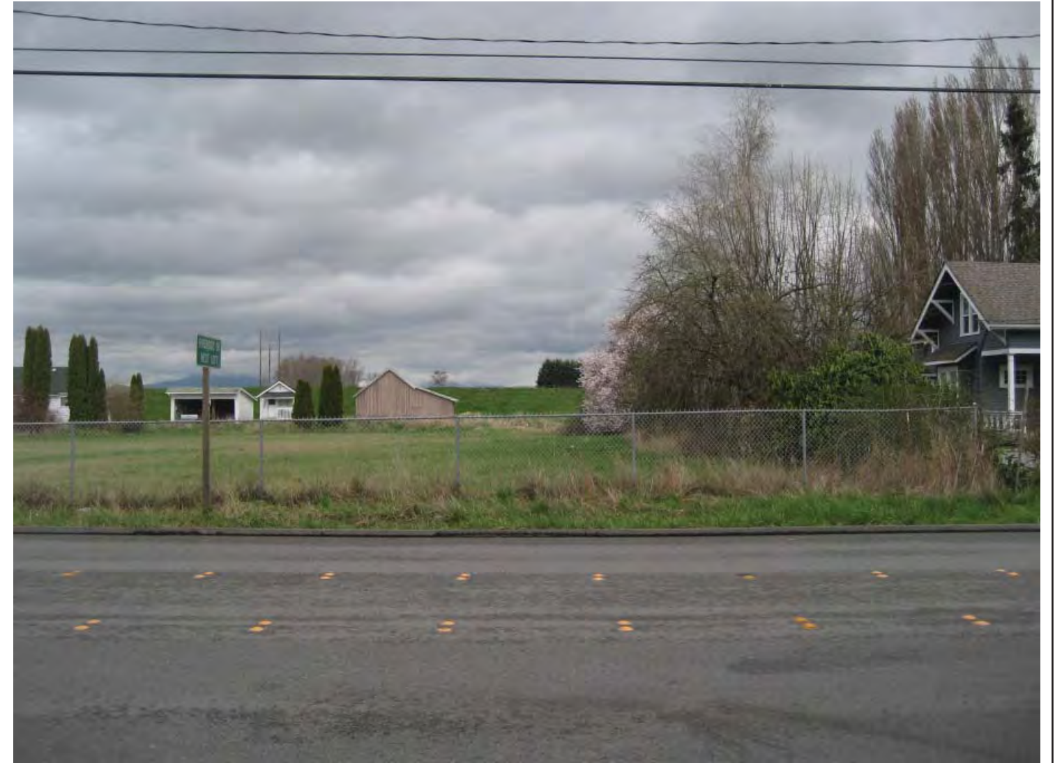
View North from Intersection of West Parkway and Hoag Road: Improved Existing Levee Alignment Alternative
