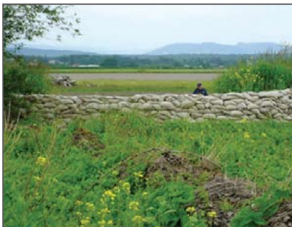
Stillaguamish River, sea dike emergency repair.
