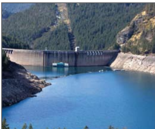
Ross Lake Dam, Upper Skagit River
